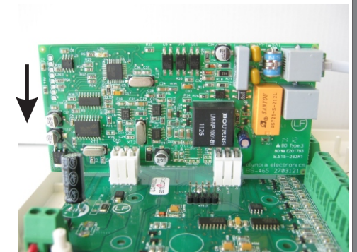
Figure 2 : Installing a BS-465 on the BS-468 panel
